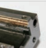
Inspection interval 3: Lubricant residue
